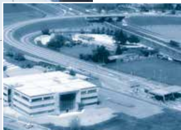
GAPI GROUP HeadQuarter - Italy
